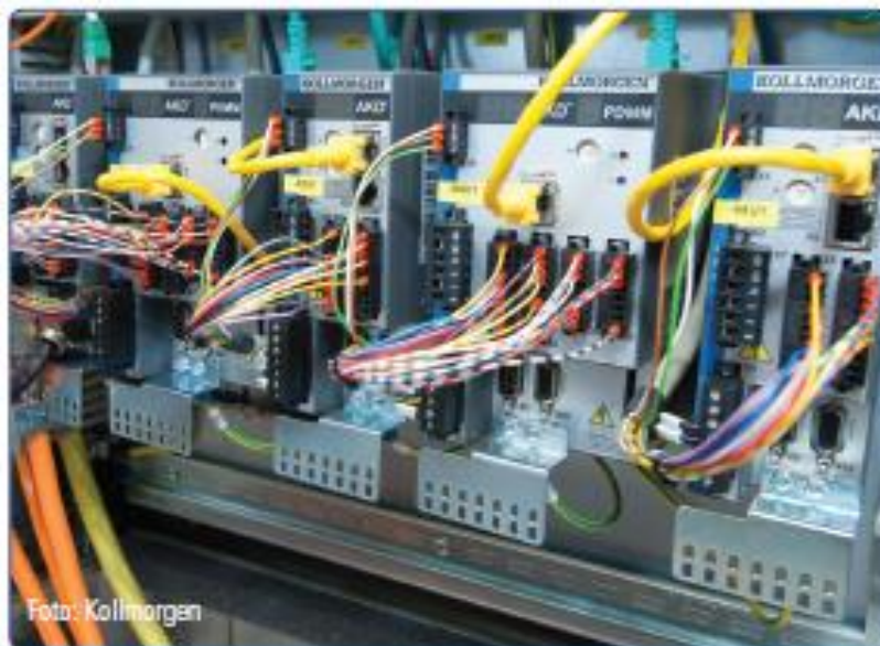
The intelligent servo inverters from the AKD PDMM range offer the computing power of an "IPC inside". At Schleuter, communication takes place via EtherCAT.
